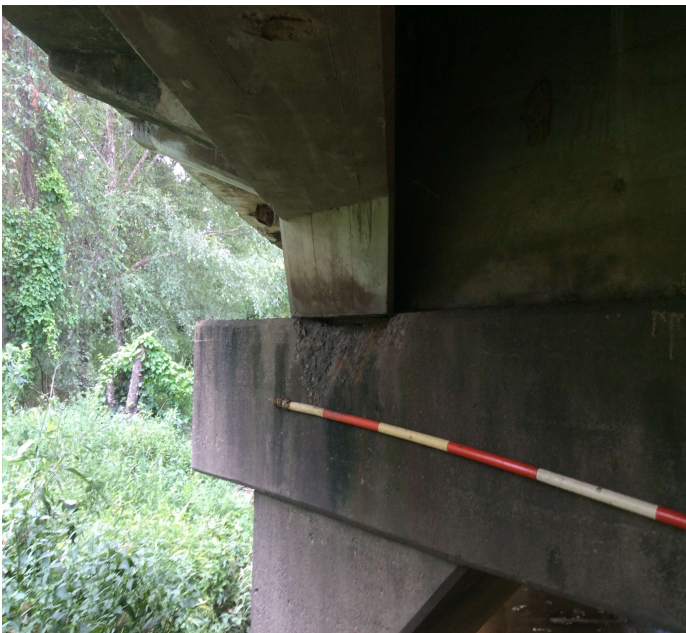
PHOTO 1 Description Bent 3, ahead side under girder 3. Spall with exposed rebar.
