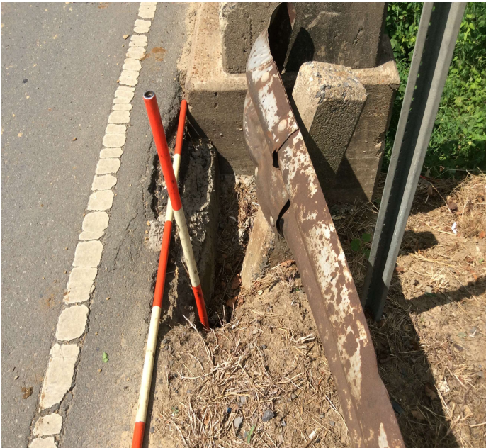
PHOTO 1 Description The approaching roadway southbound at bent 4 has deep hole and Void under the pavement. The embankment had eroded causing the approach rail to settle.
