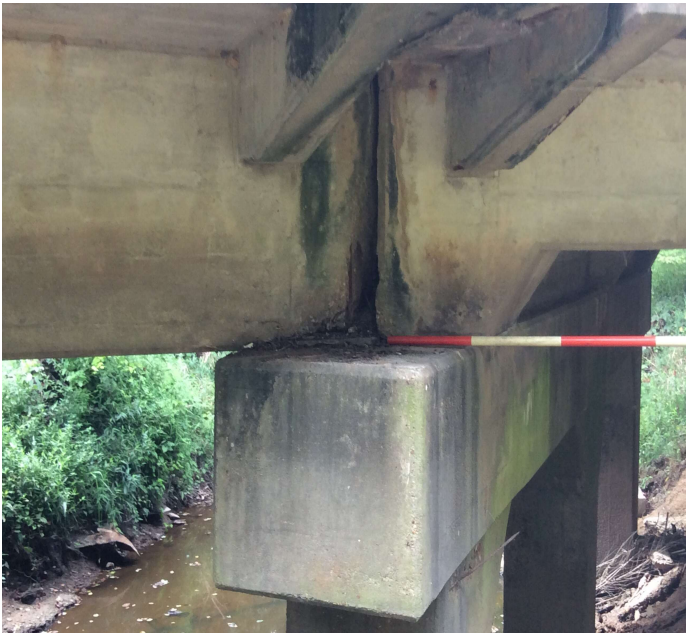
PHOTO 1 Description Bent 2, looking at the left end. Girder 1 of span 2 has a spall at the end over the bearing.
