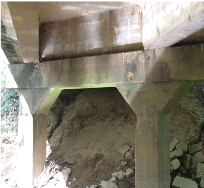
PHOTO 1 Description Bent 2, looking back. The cap has delaminations under girder 2 and a spall with exposed rebar under girder 3
